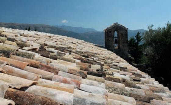
with historic tiles. The project relied on traditional regional building methods – using cypress trees as timber for the ceiling beams from an area nearby, applying traditionally manufactured lime-based mortar, and reusing original tiles when possible, supplementing them when necessary with tiles salvaged from ruins in the region.
