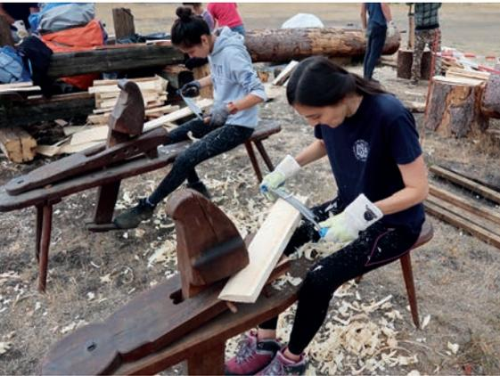
Then you start using a drawknife to finalise the shape of shingle into the ideal proportion, careful to craft a straight surface, without spikes. Master Kai taught us how to feel the surface of a correct shingle and how to replicate it through shaping. The best shingle is one that does not have branch nodes and tissues breaks, which means that the natural structure of the tree is not damaged. Meanwhile machine-made shingles last only for ten years and soon start to rot; correctly handmade
